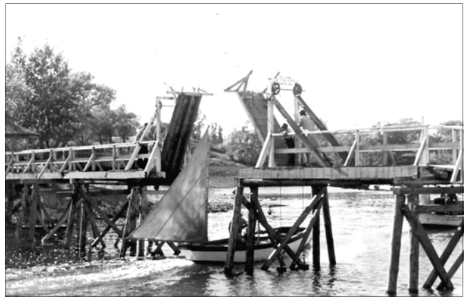
The Perkins Cove footbridge, September 1941, with dory passing through. This unique drawbridge was hand cranked by the Harbor Master and willing helpers. (Photo by David O. Woodbury)
